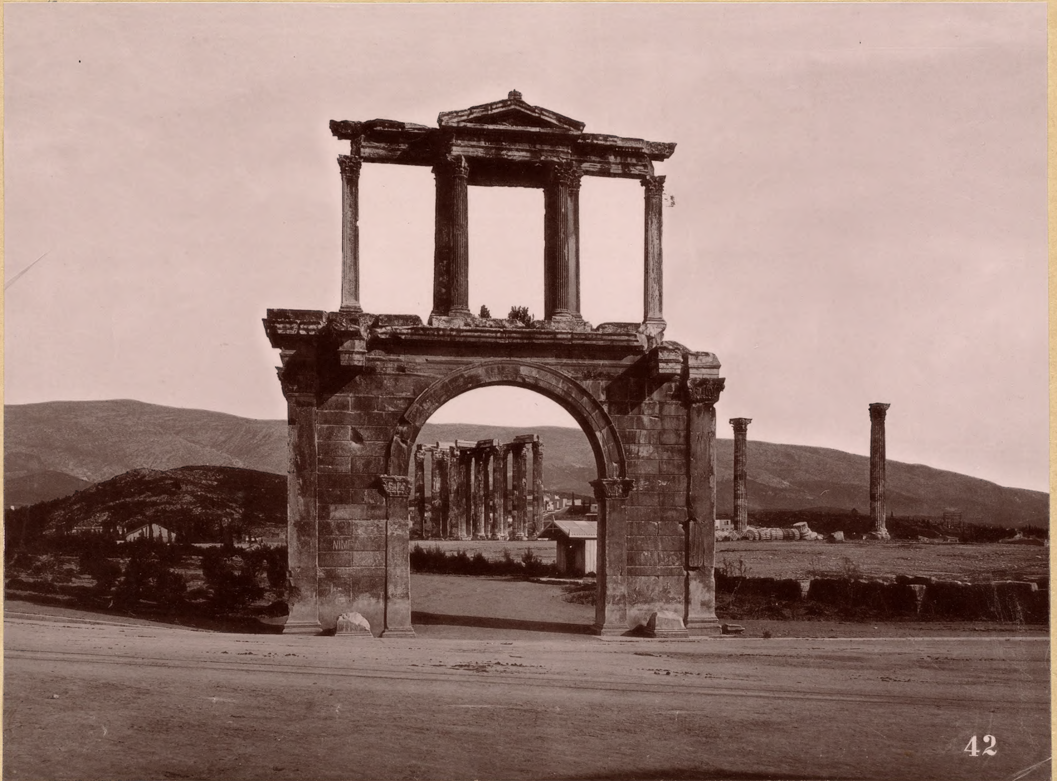
NEARER CIRCLE. EAST. ARCH OF HADRIAN. 59 ft high. 44 ft wide. archway 20 ft wide. Separated Greek City of Theseus from Roman City of Hadrian.
